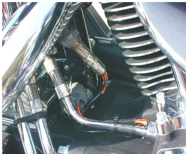
Figure 26 – Typical Sensor Installation
