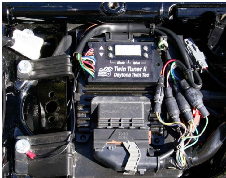
Figure 7 – Completed Twin Tuner II Installation
