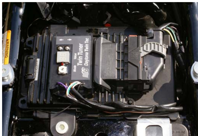
Figure 8 – Completed Twin Tuner Installation
