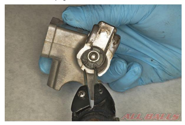
Install the snap ring with snap ring pliers. Make sure the snap ring is fully seated in its groove.
